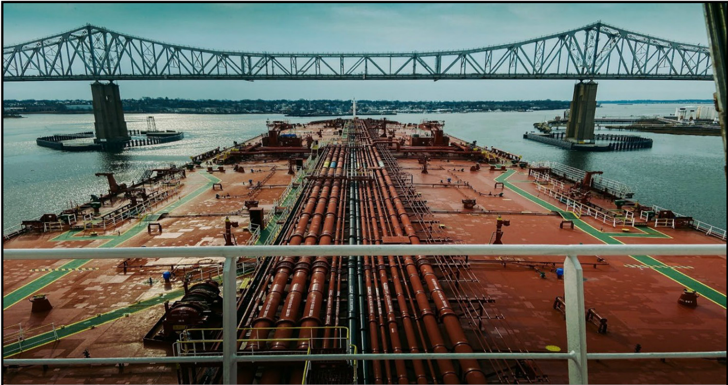
Tank Vessel transiting the Arthur Kill under the Outbridge Bridge.
